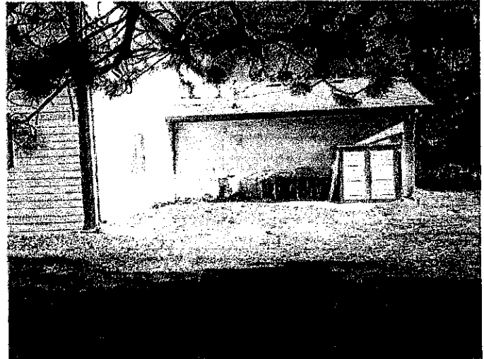
REAR VIEW (Westerly Northwesterly face of house)
